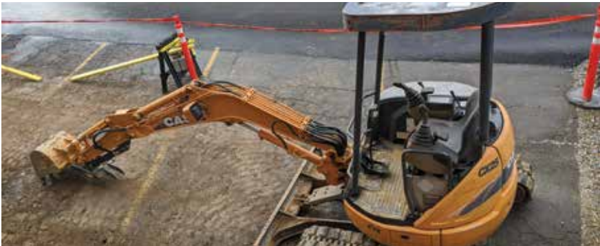
New Water Main Winter 2020
